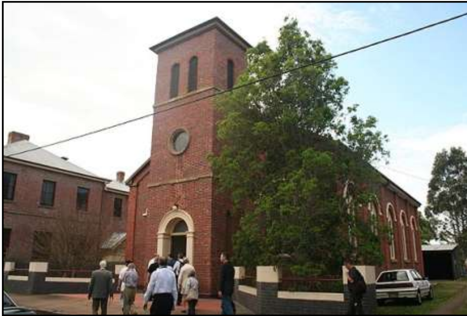
Scots' Presbyterian Church, Maitland (formerly PCEA) built 1849
